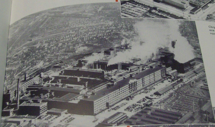
The Jefferson Plant background, where Chrysler cars are assembled. This plant also makes engines for DeSoto and Chrysler cars, and is headquarters for the Marine and Industrial Engine Division.
